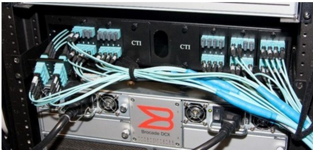
Figure 25: Device-to-Patch-Panel Trunk Cabling
