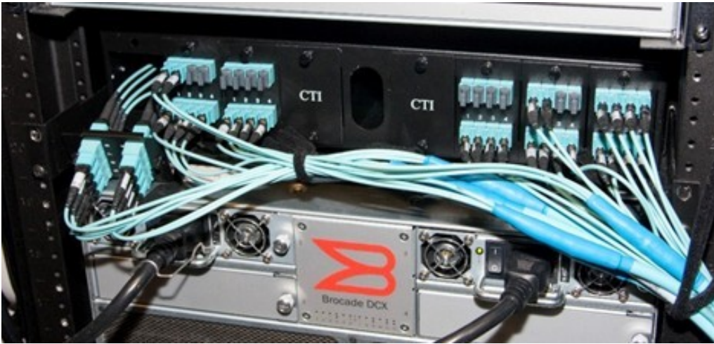
Figure 36: Device-to-Patch-Panel Trunk Cabling
