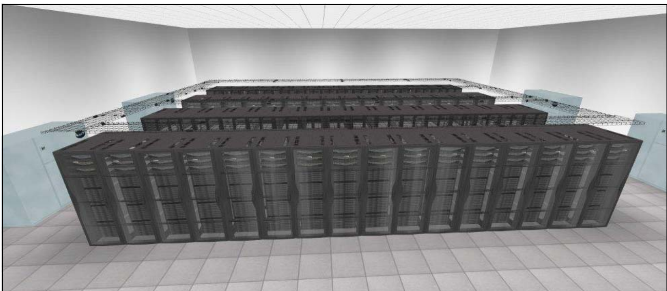
Figure 4: Pod with 2560 Servers, 64 Racks of 40 Servers Each (Source: Panduit)
